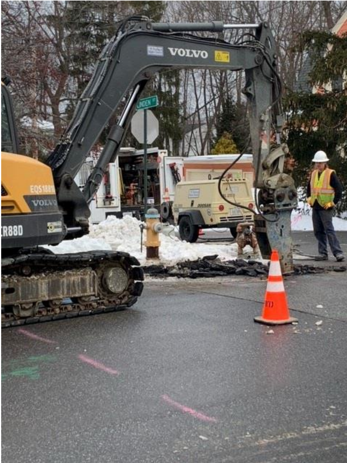
Crews repairing water main break in Portland
